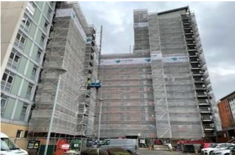
Phase1 and 2 scaffolding
