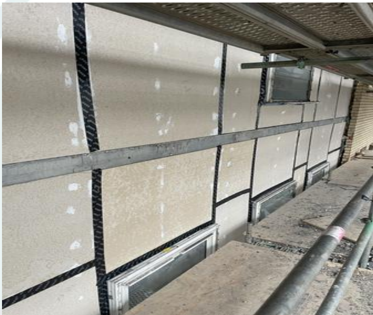
Phase 2 Y wall panels
